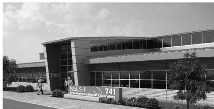
Brookhaven National Laboratory, National Synchrotron Light Source II (NSLS-II) and Lab Office Buildings.
